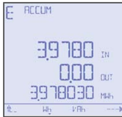
Energy in, out, total display
